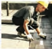
FLAT TOP ROOF
