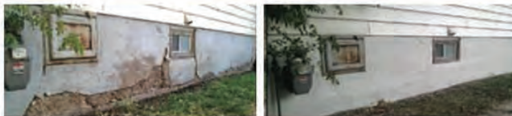
FOUNDATION REPAIRS BEFORE & AFTER
